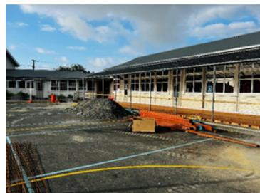
The old fence has been removed and new drainage installed. The concrete will be poured this weekend.
