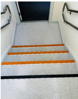
Stairs both inside and out have been capped and a handrail installed in the double block.
